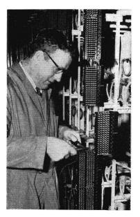
Installation of equipment for the new P.O. Room is still proceeding. Leading Hand Automatic Sub-station Electrician E. McConville is shown making one of the half million or more connexions on the 35 ft.-long wiring frame that was manufactured by Bendigo Workshops.
