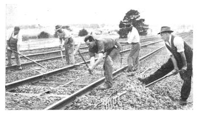
No. 10 gang (Ganger F. Law) are replacing a sleeper on down side of station.
