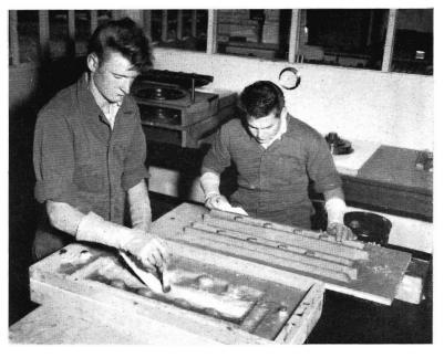
Patternmakers at Newport Workshops use epoxy resin and fibre glass to make a mould.
