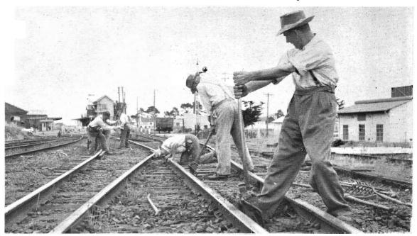
At up end of station, No. 9 gang (Ganger C. A. Vallence) lift crossing for replacing timber.
