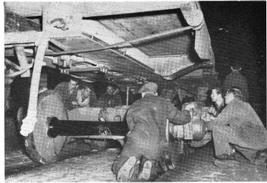
Placing bogie in position under wagon.
