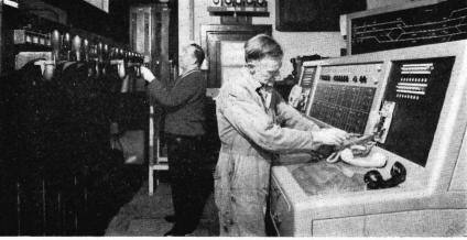
In the Camberwell signal box, the new scheme, with its enlarged track layout, necessitated replacing the old electro-mechanical interlocking machine with a new route type, push-button console. Picture shows an electrical mechanic installing the new console (*right*). The old machine (*left*) was installed forty years ago.
