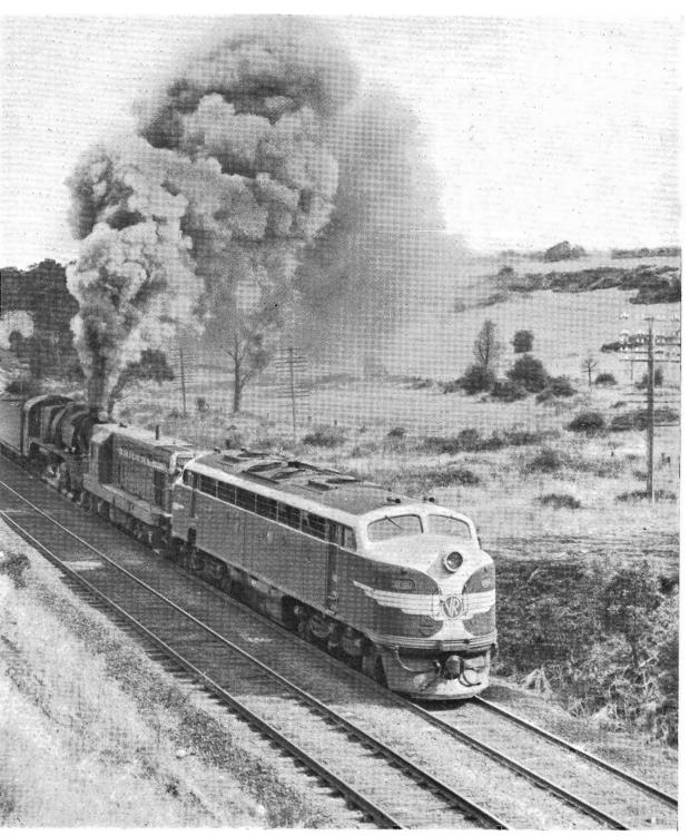
d harvest, movement of grain that was in excess of country storage capacity was completed before the end of last month. Picture shows a wheat train being hauled up the Warrenheip bank by B and T class diesel-electrics and R class steam locomotive.
