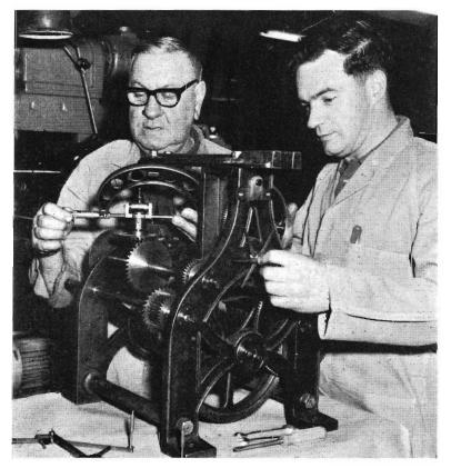
Electrical Fitters W. Clifton (*left*) and E. Roberts at work on the clock mechanism at the Electrical Depot Workshops
