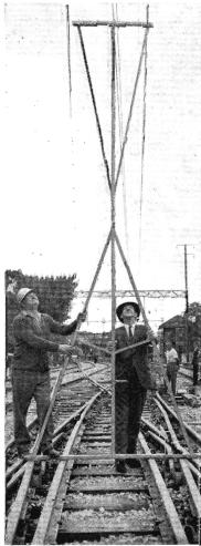
At Hawthorn, overhead staff check the stagger of the contact wire. The staggering prevents uneven wear of the contact strip on the pantograph.
